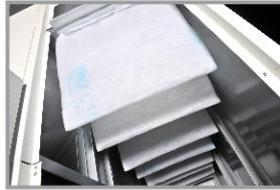
Air intake prefiltering. Honeycomb pocket filters.
